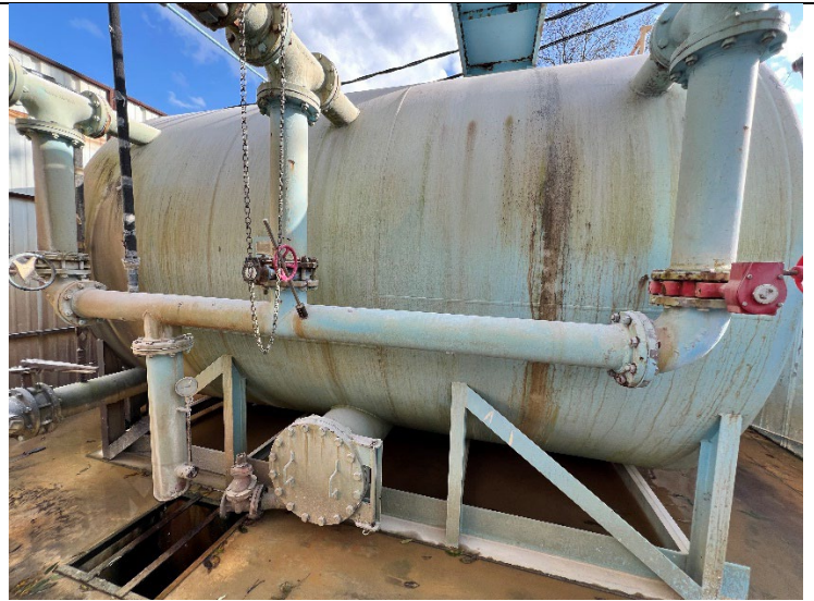
Figure 20: Pressure Filter #2
